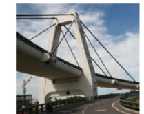
Bridge Abutments, Pillar Piers & Footings
