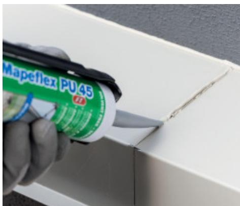
*Flexible sealing of construction joints*
